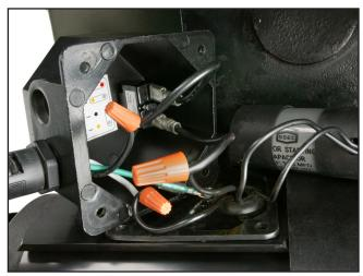
Figure 61. Motor junction box wiring.
